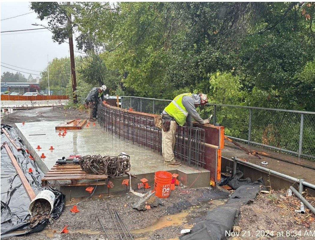
Figure 10 – TPS placing Barrier Rebar in the rain.
