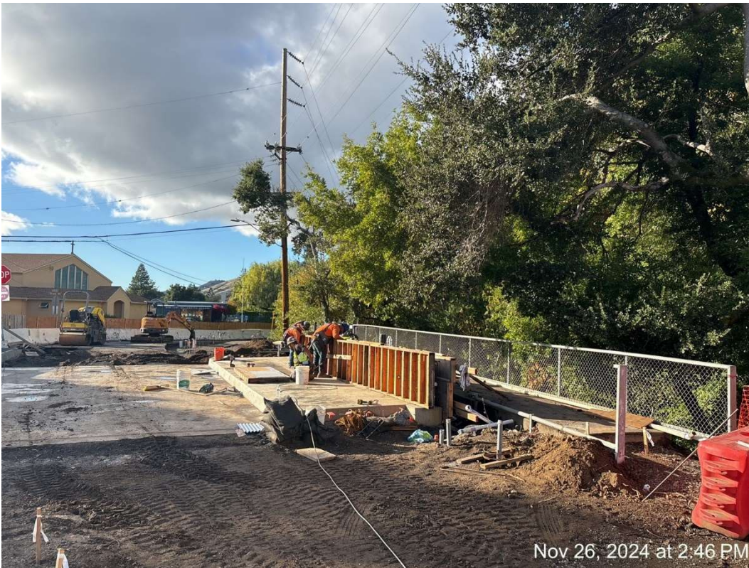
Figure 13 – Bridge Barrier Formwork.
