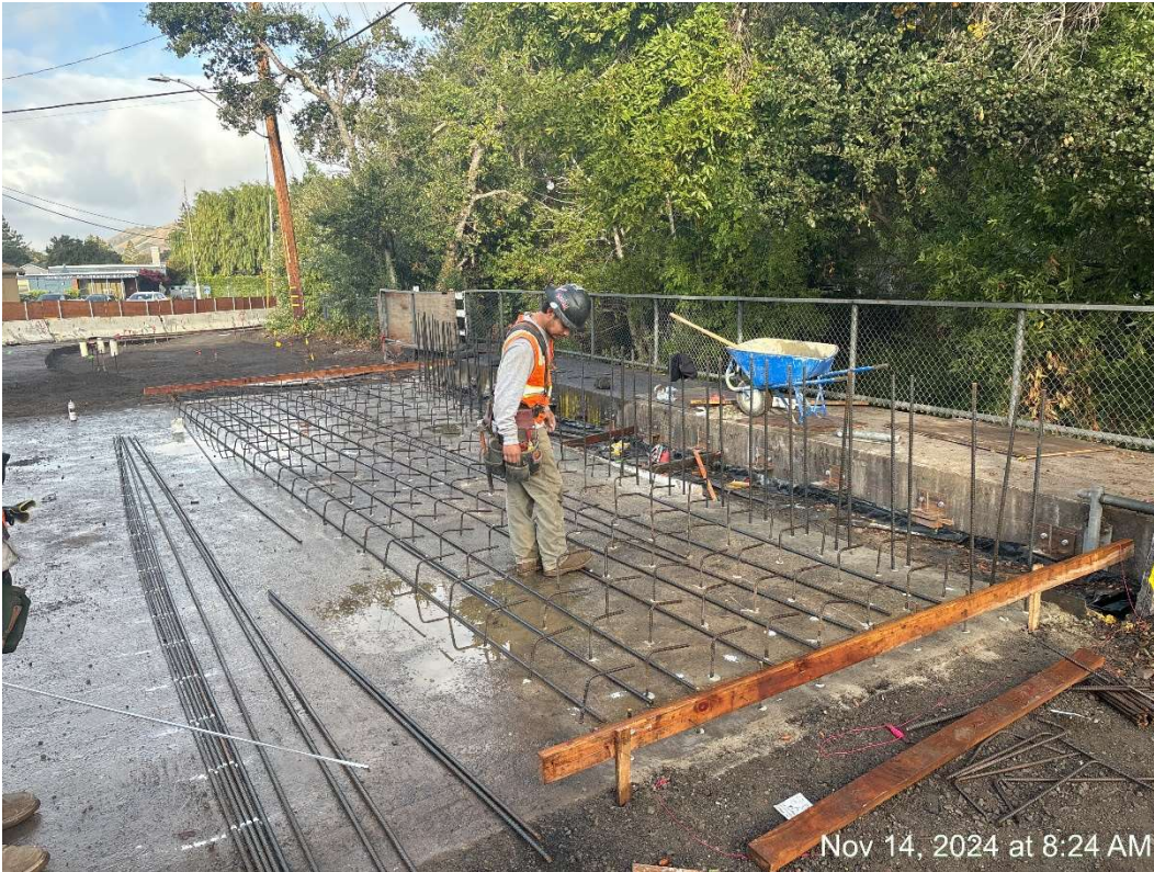
Figure 3 – Sidewalk and Barrier Rebar.
