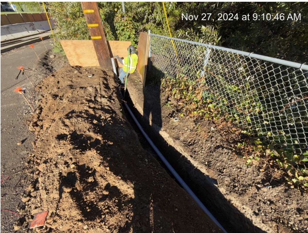
Figure 14 – Electrical contractor digging PG&E Trench to service meter.
