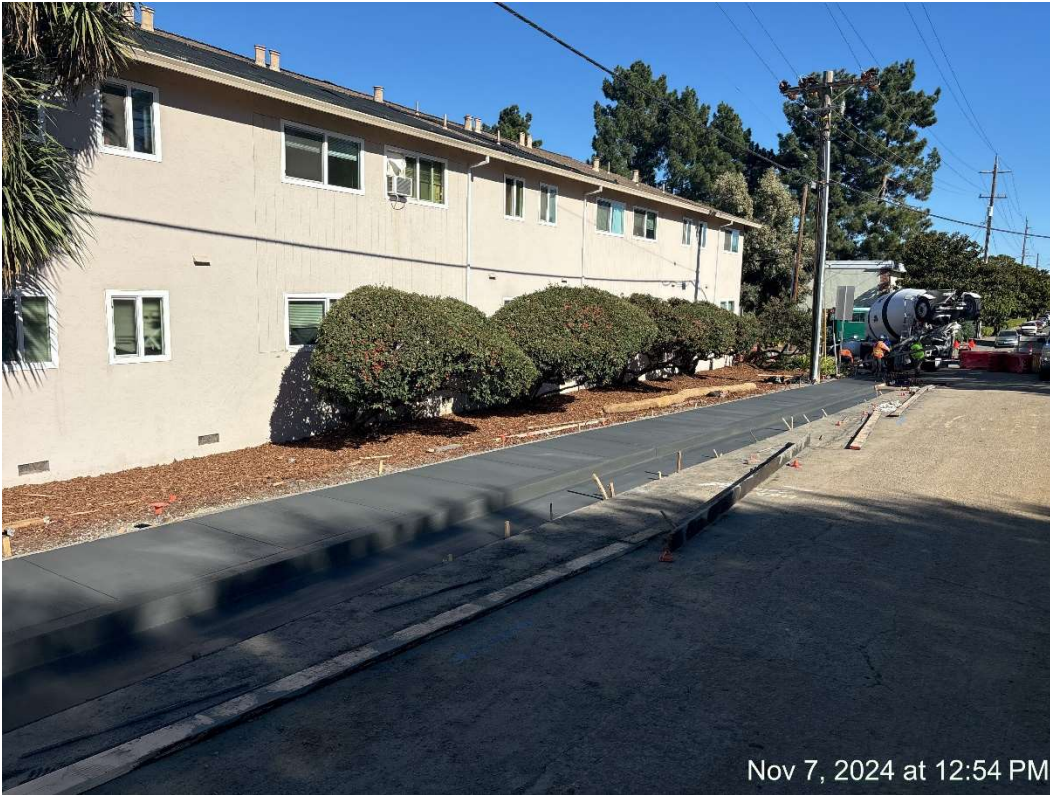
Figure 5 – Poured Sidewalk, Curb & Gutter.
