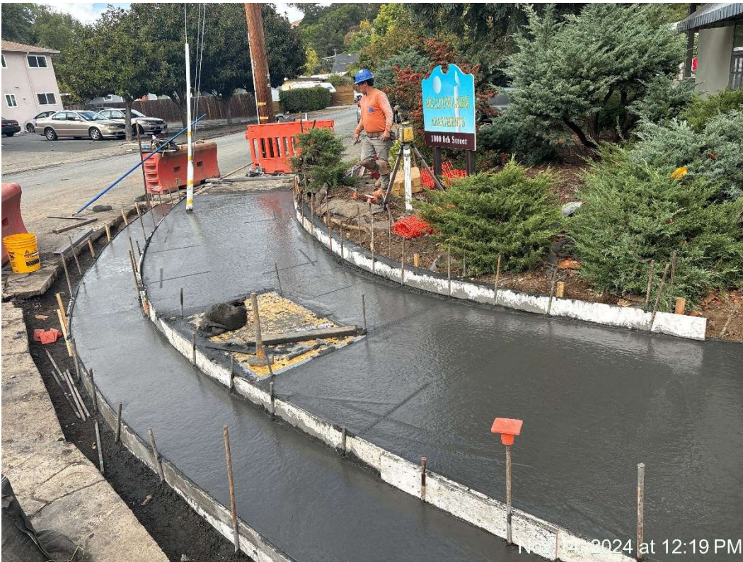
Figure 9 – Poured ADA Ramp – NE Corner of Grant Ave & 8 th Street.
