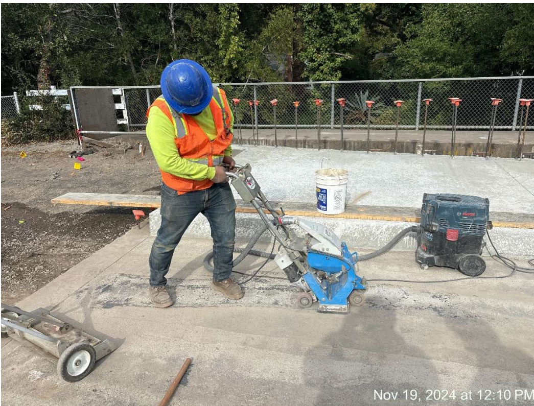
Figure 8 – Shotblasting bridge deck.
