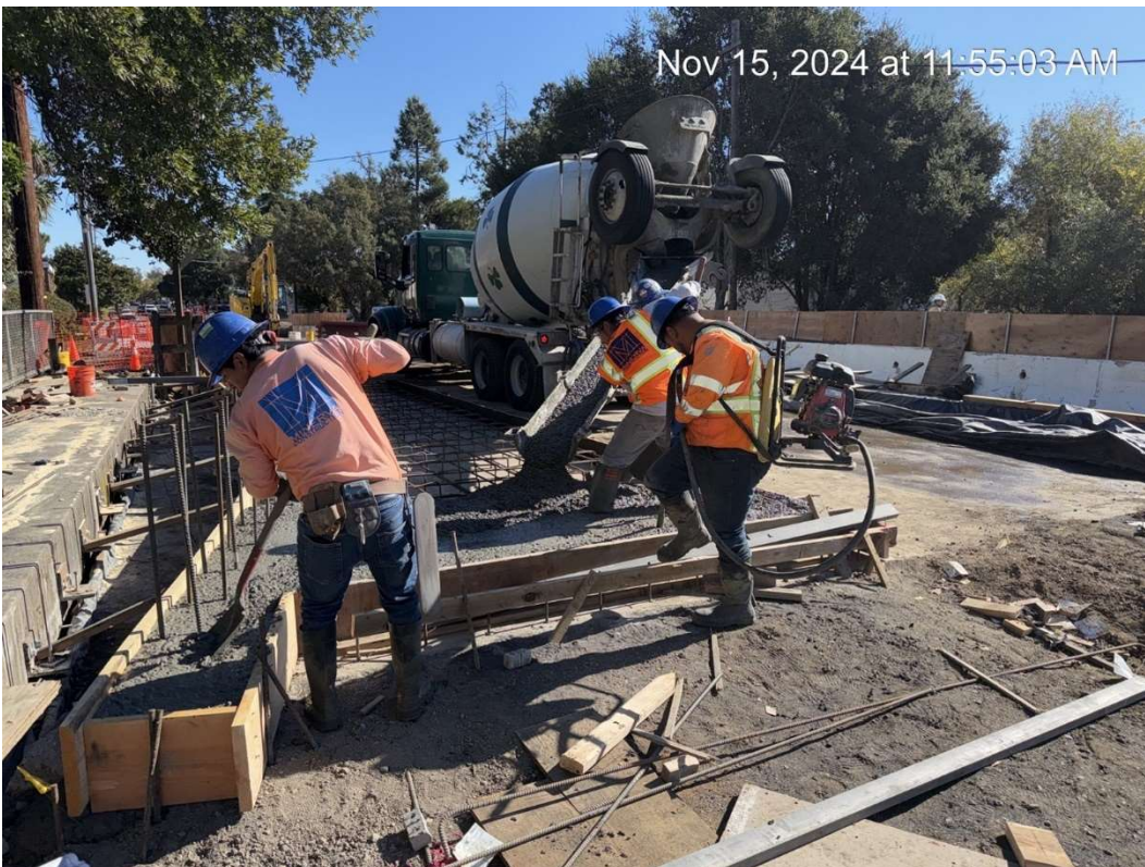
Figure 4 – Pouring bridge sidewalk.
