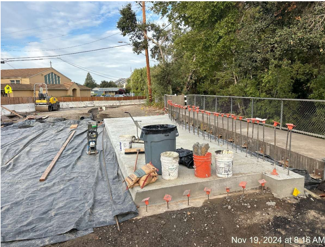
Figure 7 – Sidewalk Poured and complete.
